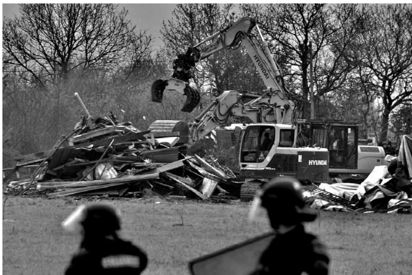
The first of 29 houses demolished by the police at ZAD in April 2018.
